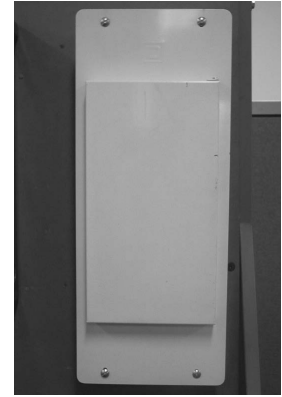
Step #4 Complete Installation
